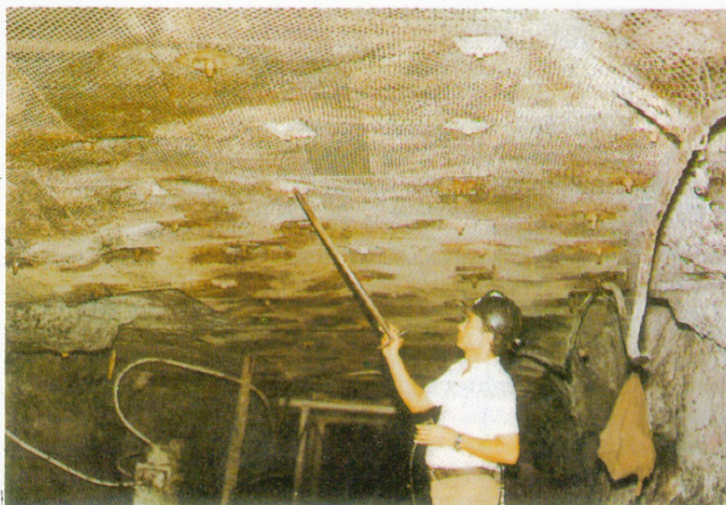
Combination of wire netting and roof bolting
