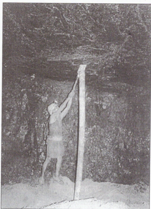
Dismantling of fly-ash props
