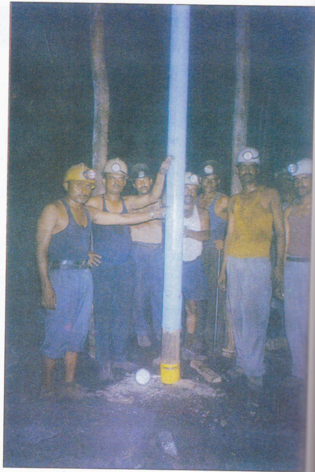
Rigid pit prop mounted on a load cell installed in underground workings
