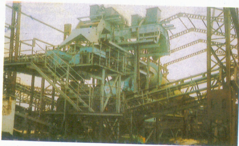
Pilot plant. incorporating barrel washer
