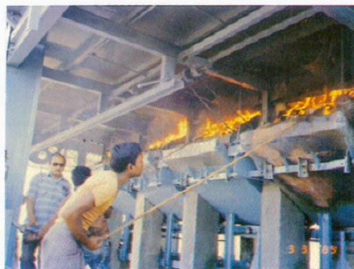
Retorts in operation
