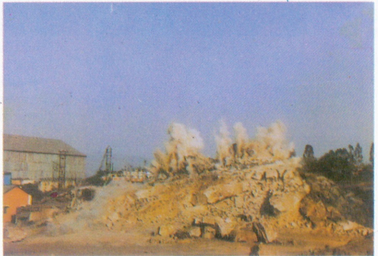
Blasting near surface structure
