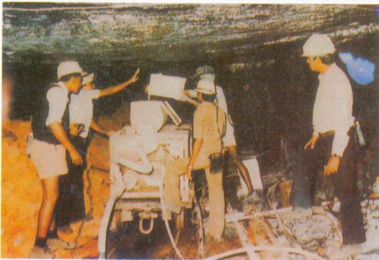
Spraying machine - charging of sealant
